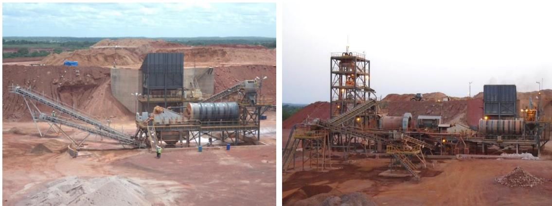
Figure 3 – Comminution Circuit - Before and After Phase 2 Expansion
